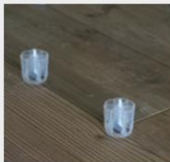
T-shaped leveler installation.
