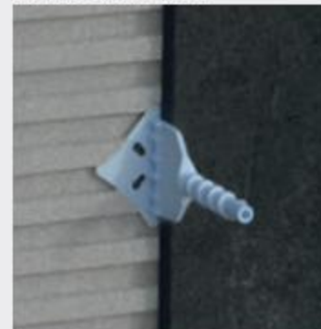
Linear leveler installation.
