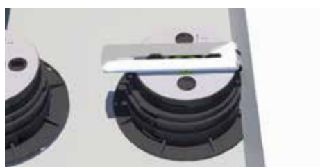
16. Position the SUPACLPP spacer clip.
