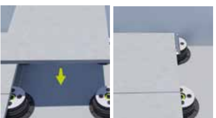
7. Install the tile.
